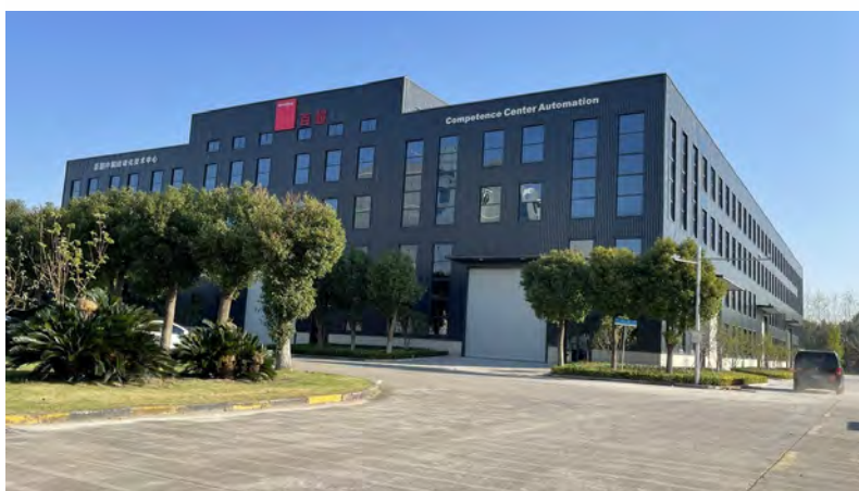
The new Competence Center Automation in Shanghai (China) for automation solutions.
